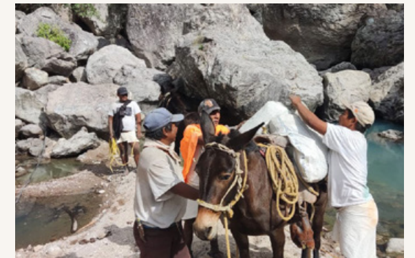
Community members transport materials for the construction of water storage tanks
