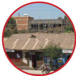
With a focus on "Champion Villages," local partners are installing small-scale water supply and sanitation infrastructure
