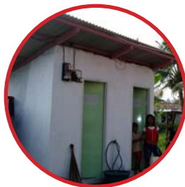
To actively support hygiene and sanitation practices, new public latrines were installed in Kampung Wangkal
