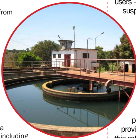
Renovating a dilapidated water treatment system provides clean water for 25,000 residents of Chimoio
