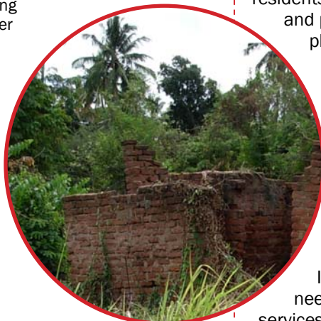
Replacing unusable sanitation infrastructure will help alleviate stresses on valued water resources
